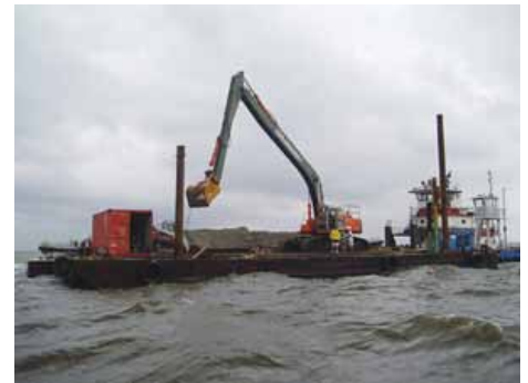
Barge with heavy machinery begins work on oyster-habitat restoration project in Pamlico Sound.
