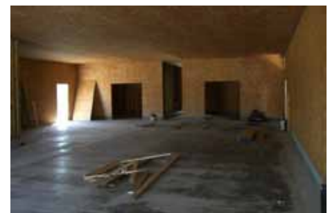
Top: Aquaculture Center nearly complete. Bottom: Interior awaits installation of saltwater equipment for aquaculture research.
