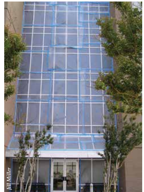
Repairs in progress at CMAST. Left: Workers in cherry pickers caulk and seal all windowsills. Right: Windows were masked on the entire structure before waterproof spraying could begin.
